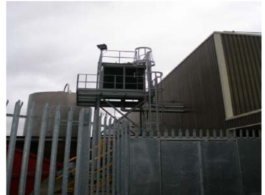
Tower location on site
